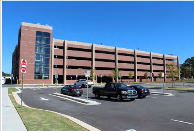
Forsyth County parking deck
