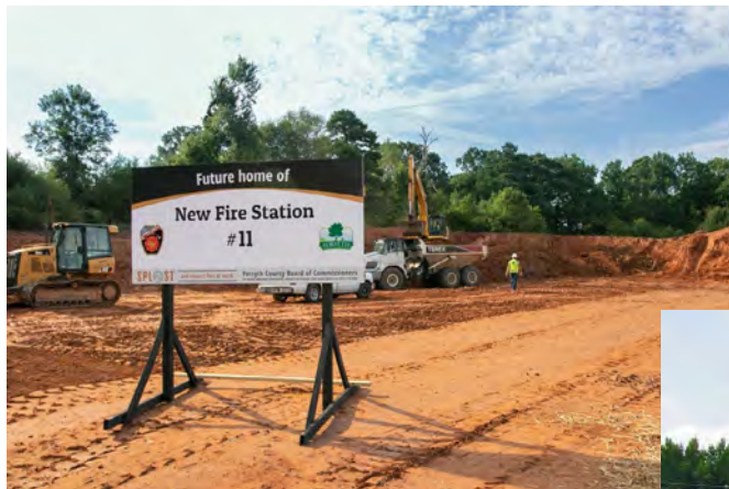
Future site of new Fire Station #11 funded by SPLOST
